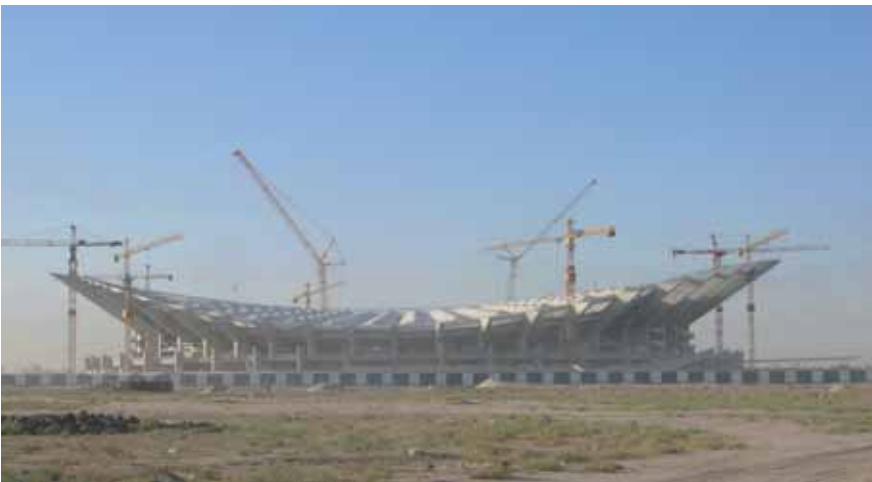
Al Sheik Jaber Al-Ahmad Stadium, Kuwait Lifting and tensioning of a fully-locked cable roof structure by 32 units with a total pulling capacity of 10,560t.
