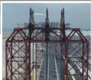
Detail: top of a temporary lifting tower
