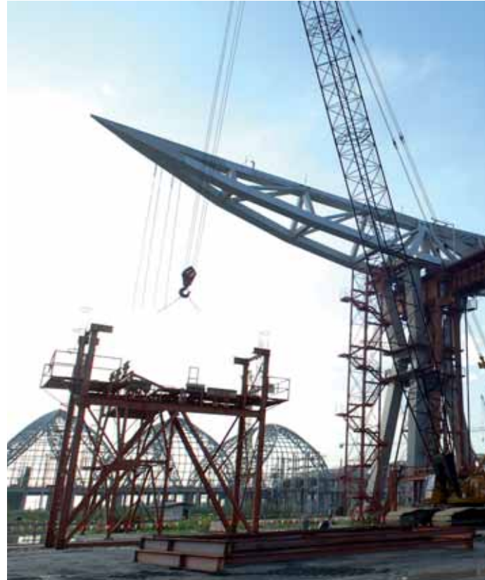
Suvarnabhumi International Airport, Bangkok, Thailand Lifting and positioning of 210m-long giant 'super trusses' weighing between 1,600t and 2,200t. Lifting height: 25m
