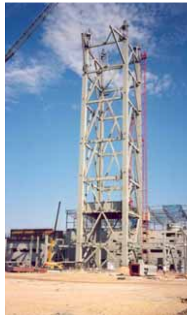
Afsin Elbistan B 4x 360 MW PP, Turkey Lifting of 520t suspension grillages to a height of 120m. Total weight of structures lifted in the four boiler houses: 10,000t
