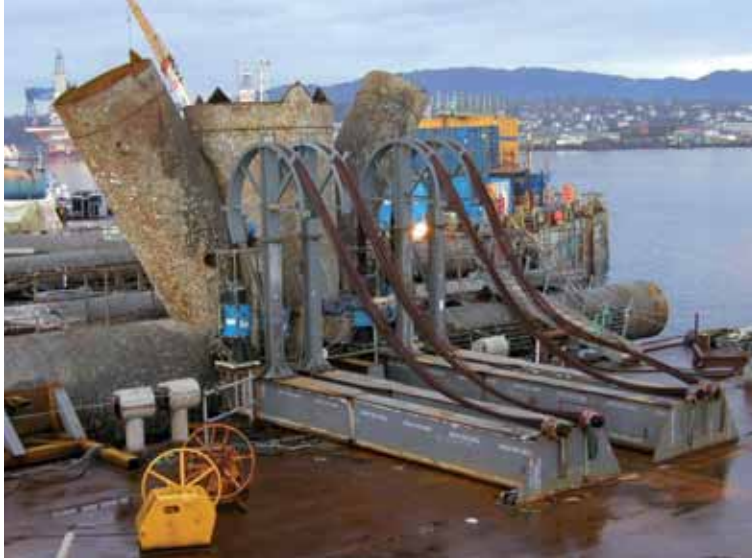
Maureen Alpha Platform decommissioning, Stord, Norway Skidding of a 12,000t deck by 90m onto the wharf. Lifting of storage tanks and lattice substructure for dismantling. Platform base area: 7,800m 2 .; height: 235m; weight: 105,000t
