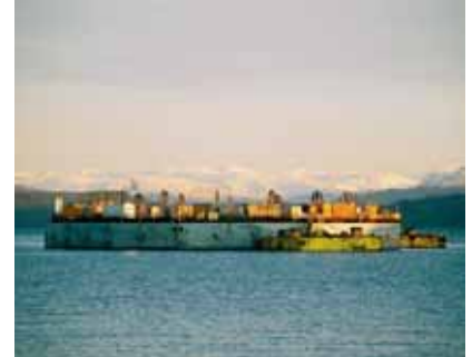
Maureen Alpha Platform decommissioning, Stord, Norway Skidding of a 12,000t deck by 90m onto the wharf. Lifting of storage tanks and lattice substructure for dismantling. Platform base area: 7,800m 2 .; height: 235m; weight: 105,000t
