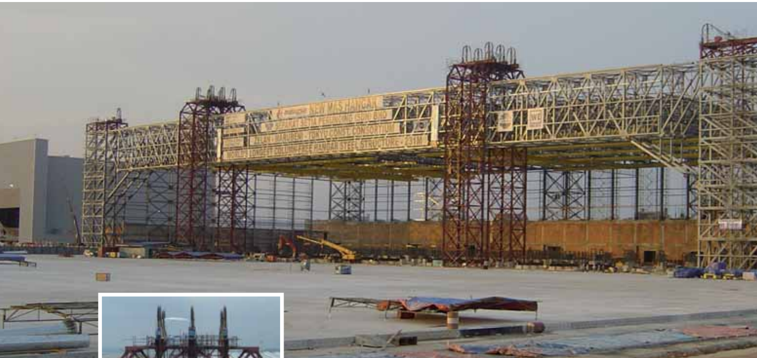
MAS (Malaysia Airlines Systems) Hangar, Kuala Lumpur, Malaysia Lifting of a steel roof structure, weighing about 5,000t and covering 22,000m 2 . Lifting height: 32m. In 2007 it became the hangar with the longest column-free span in the world.
