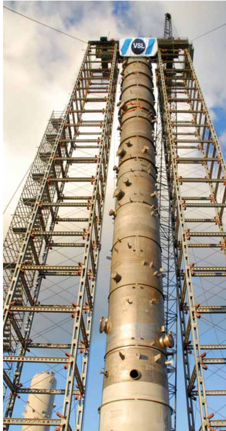
Camisea Gas Project, Malvinas Plant, Peru Lifting of two deethanizer towers, each with a height of 49m and weighing 300t.
