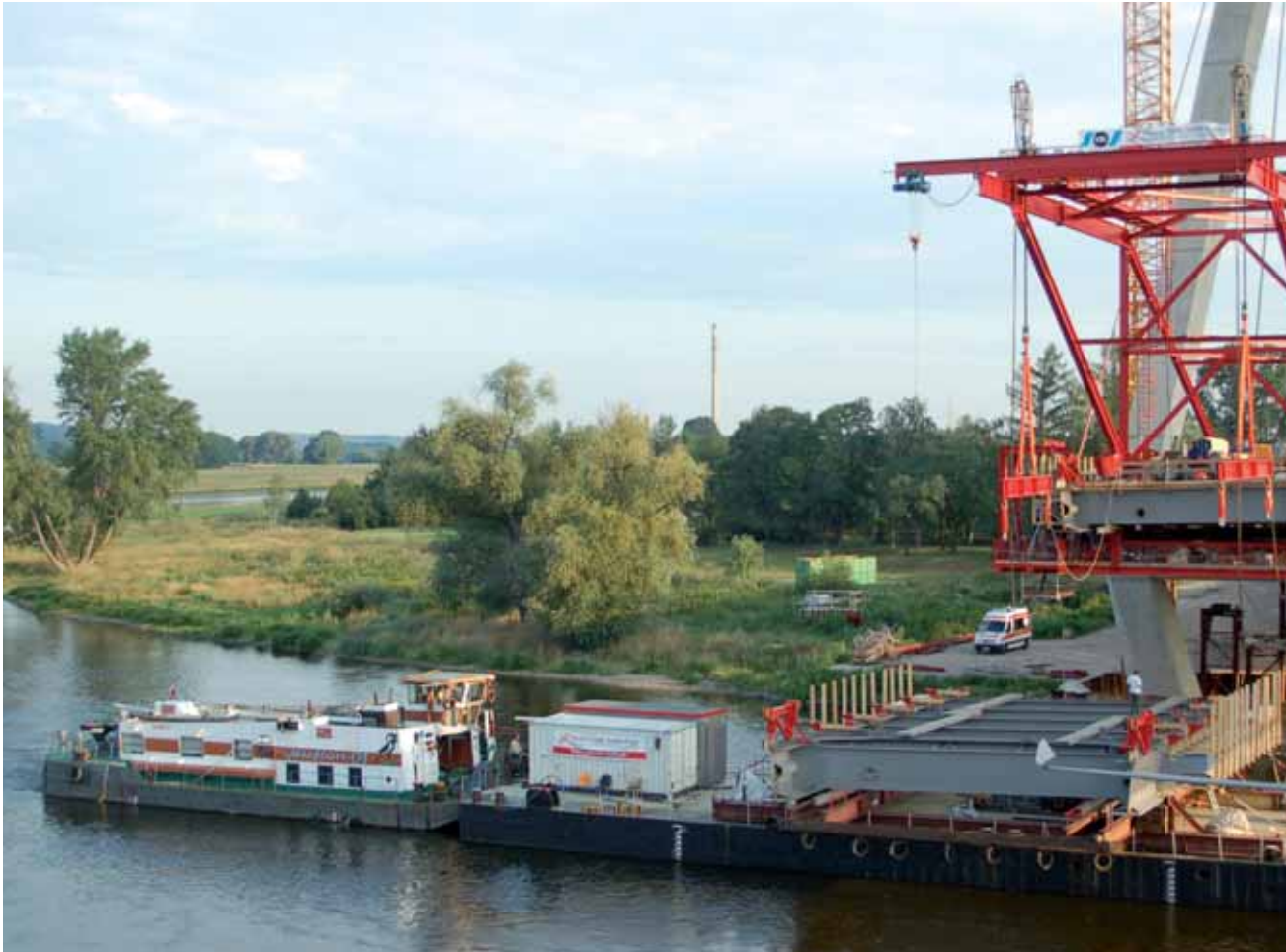
Elbebridge, Niederwartha, Germany Erection/lifting of ten 120t deck segments by 14m.
