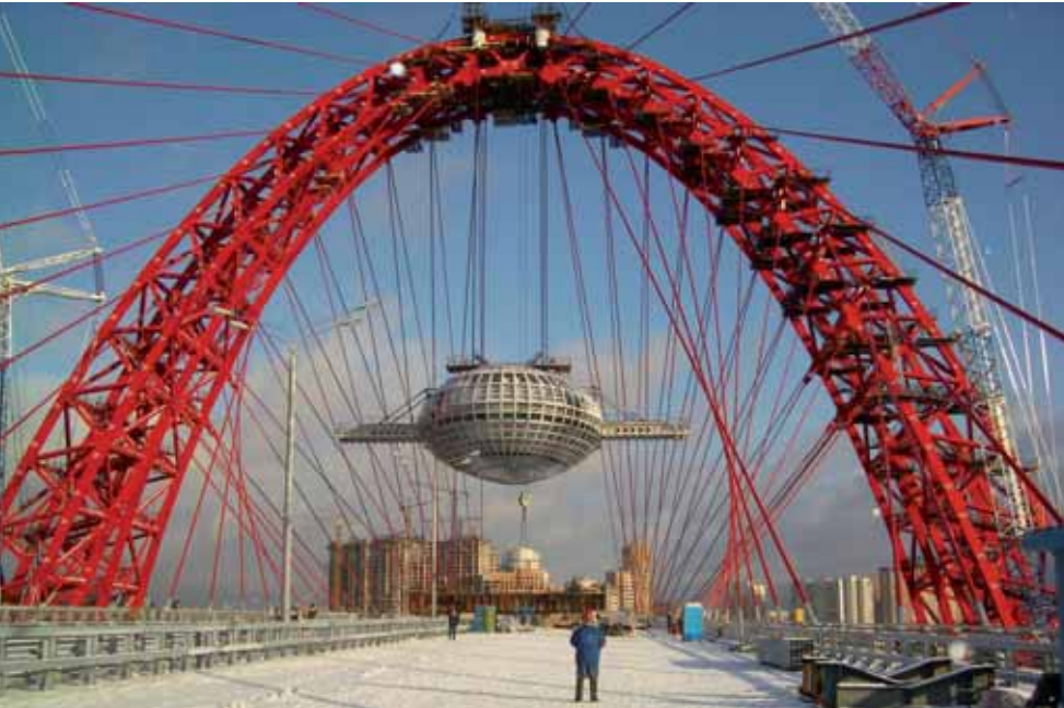
Zhivopisni Bridge, Serebryany Bor – Moscow, Russia Lifting by 55m of a panoramic restaurant with a weight of 660t
