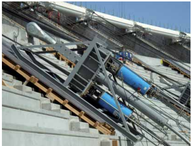
Cable roof project Lifting units with a specially-designed cradle
