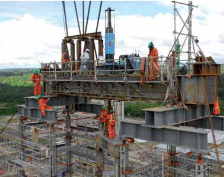
Camisea Gas Project, Malvinas Plant, Peru Lifting of two deethanizer towers, each with a height of 49m and weighing 300t.
