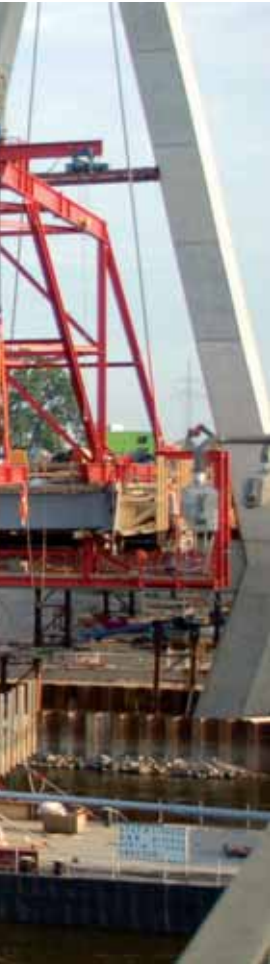
Woronora Bridge, Sydney, Australia Integrated launch and braking system, with 6.5% downhill launch of the 521m-long superstructure, weighing 20,000t.
