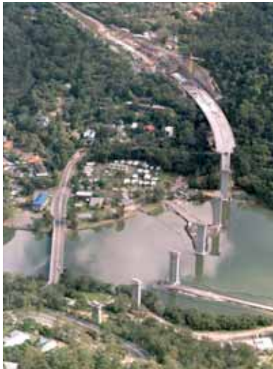
Woronora Bridge, Sydney, Australia Integrated launch and braking system, with 6.5% downhill launch of the 521m-long superstructure, weighing 20,000t.
