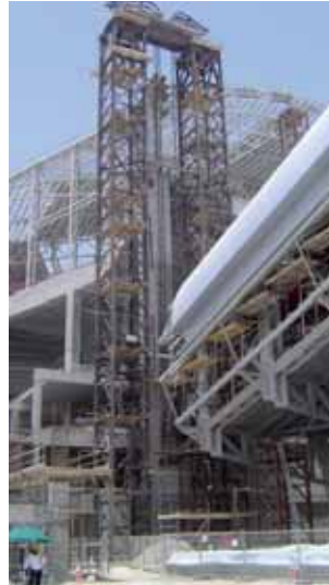
Ski Dome, Dubai Mall, Dubai, UAE Lifting of a 2,800t steel structure complete with concrete slab and partial cladding to a height of 60m to form part of a 400m indoor ski slope.
