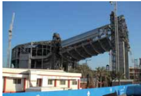
Ski Dome, Dubai Mall, Dubai, UAE Lifting of a 2,800t steel structure complete with concrete slab and partial cladding to a height of 60m to form part of a 400m indoor ski slope.
