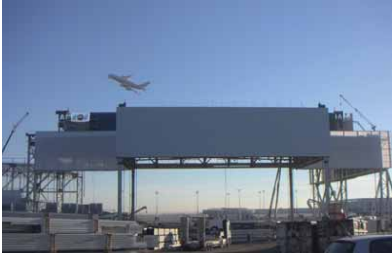
Airbus A380 Hangar "Saurous, Lagardère", Toulouse, France Lifting by 18m of four 1,700t hangar roofs.
