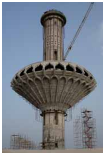
Dammam Water Tower, Damman Al-Khobar, Saudi Arabia Lifting a 8,100t concrete bowl to a height of about 60m.
